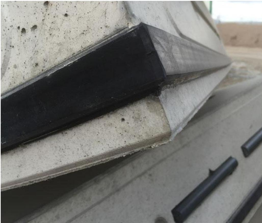
*Corner of a cast-in tunnel segment gasket*
