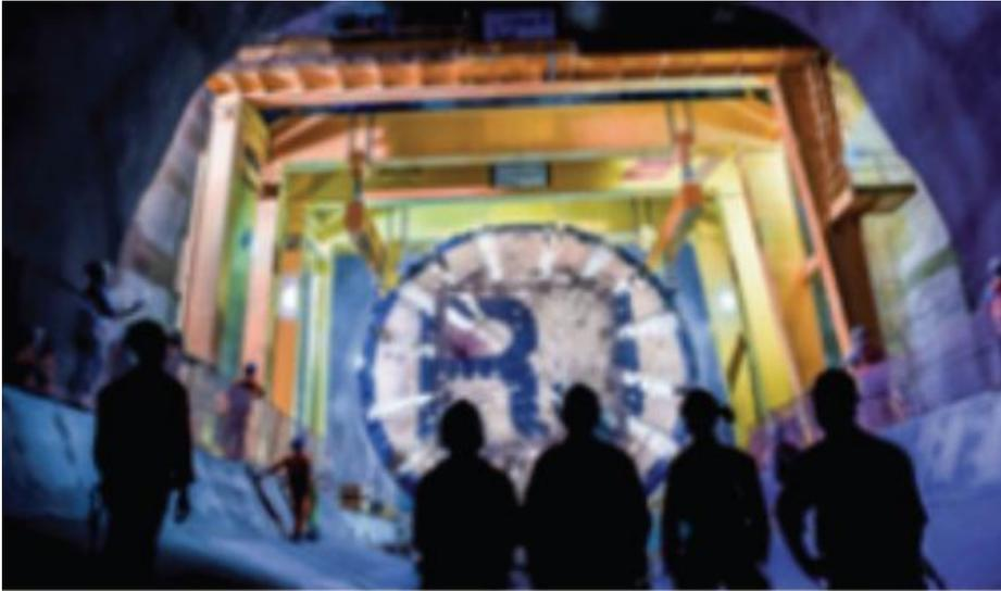
The shield-driven tunnel of metro line 4 in Rio de Janeiro (Brazil) has an approximate length of 5.2 km. the excavation was performed using a hybrid earth pressure balance shield with an excavation diameter of 11.51 m and passed through complex geology that included a long stretch of pure sand bounded by two stretches of hard, highly abrasive rock. Considerable reduction in materials, for conditioning consumables, and energy of power consumption were achieved with this hybrid EPB technology.
