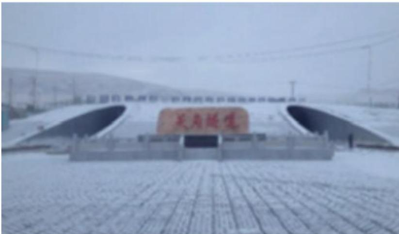
The New Guanjiao Tunnel is a key project of the second line of Xining-Golmud section of Qinghai-Tibet Railway with a total length of 32.690km. The tunnel, a two-set single-track tunnel with an average elevation of 3400m, operates with
