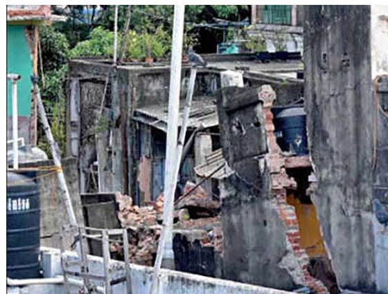
Uncontrollable ground-loss settlement caused wide spread damage and collapse of old buildings (Image: TunnelTalk)
